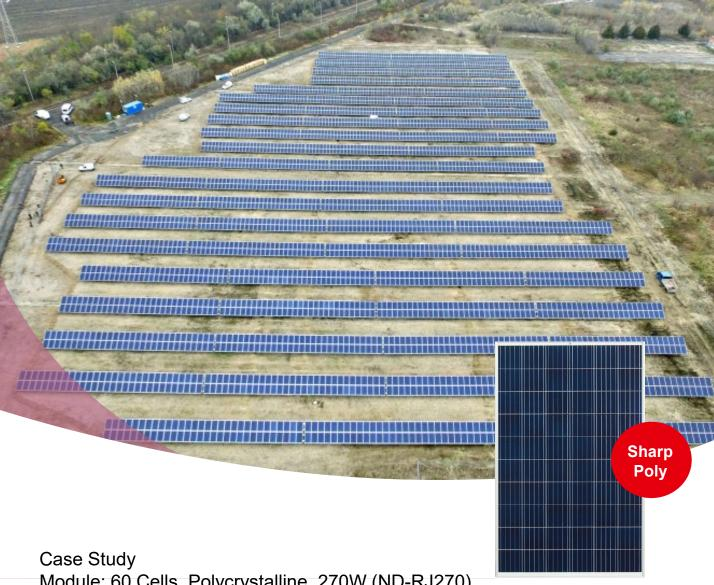
Module: 60 Cells, Polycrystalline, 270W (ND-RJ270)
